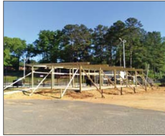
Construction continues at the city pool
